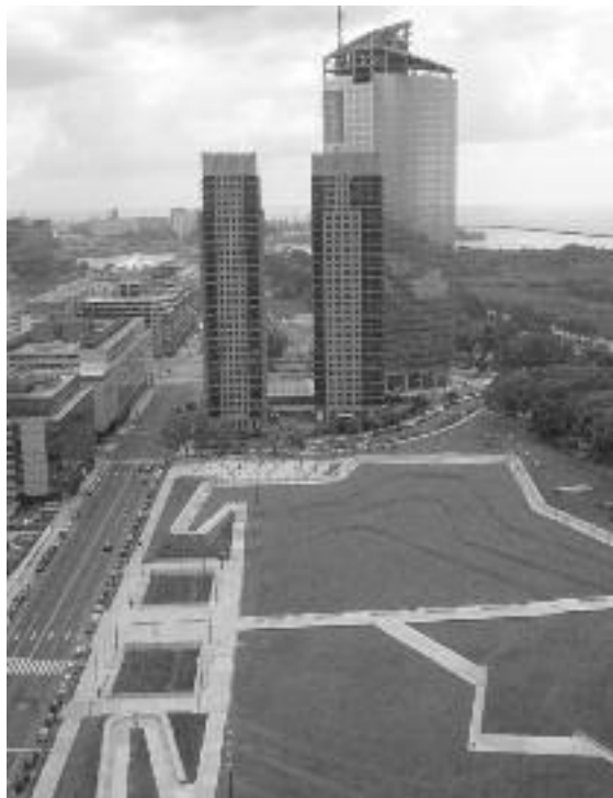
Figure 11. The corporate towers in Puerto Maderos and the Micaela Park under construction. Source: A. Arrese, 2007
