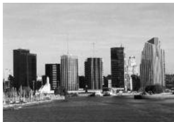
Figure 12. The Santa Catalina Towers with the Boston Bank at the end: view from the river. Source: Martin Evans
